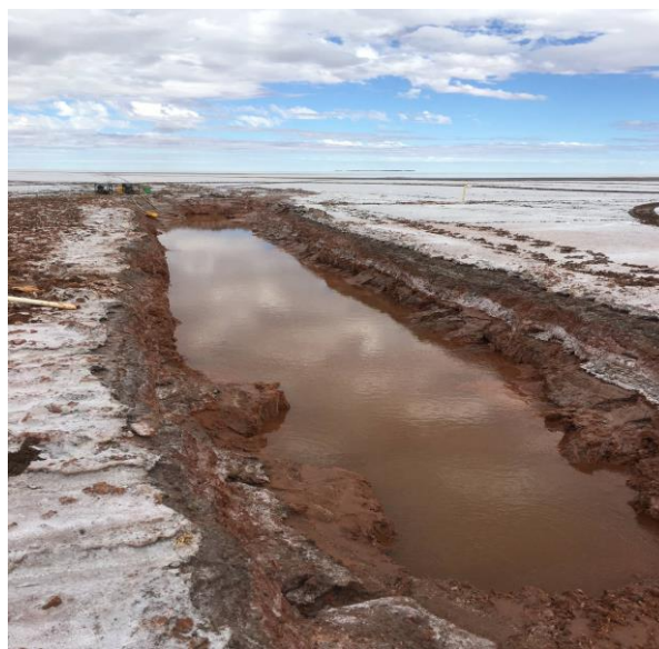
Figure 2B - Trench 10 – Steady State
