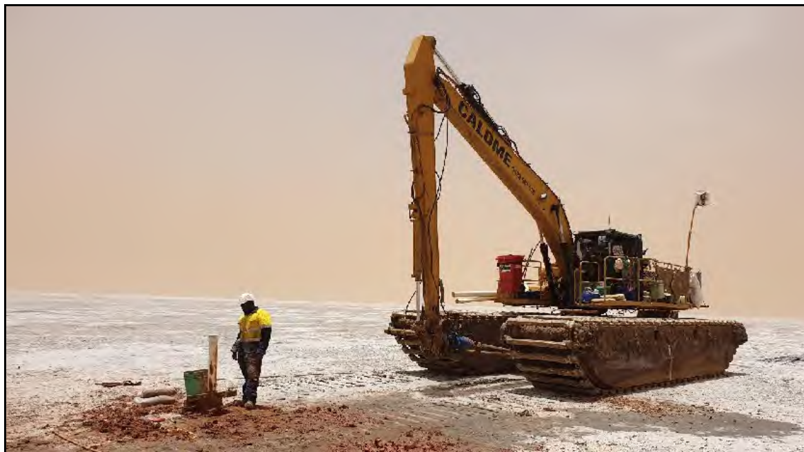
Figure 4. A completed bore
