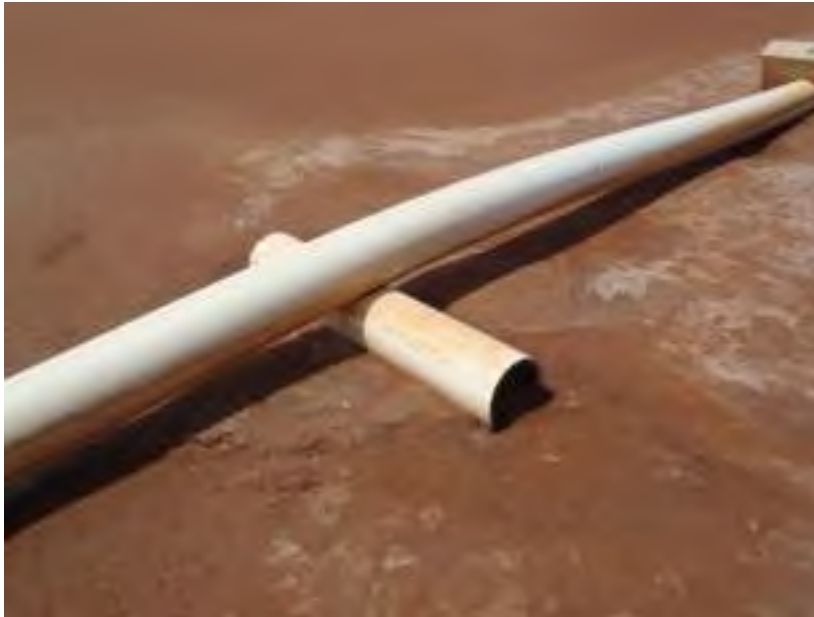
Plate 6. Raised water pipeline
