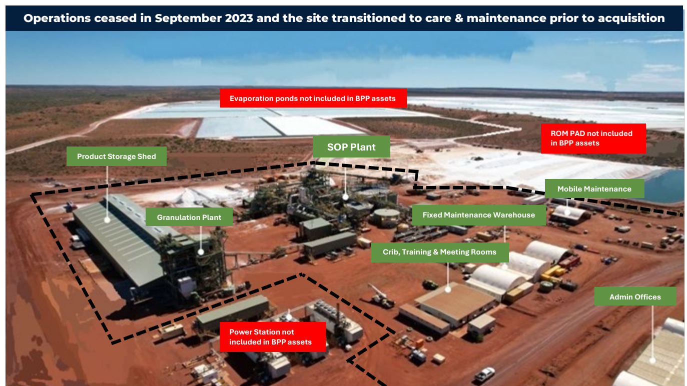
Figure 1 – Photograph of the Beyondie Potash Project in 2023 when in operation by KLL. The assets acquired comprise a fully constructed processing plant, site offices and maintenance infrastructure. Specific plant components include, KTMS crushing circuit, Kainite conversion circuit, column flotation circuit, liquor cooling heat exchangers, evaporative cooling circuit, product separation centrifuges, SOP recovery and granulation units, RO water plant and a bulk storage shed.
