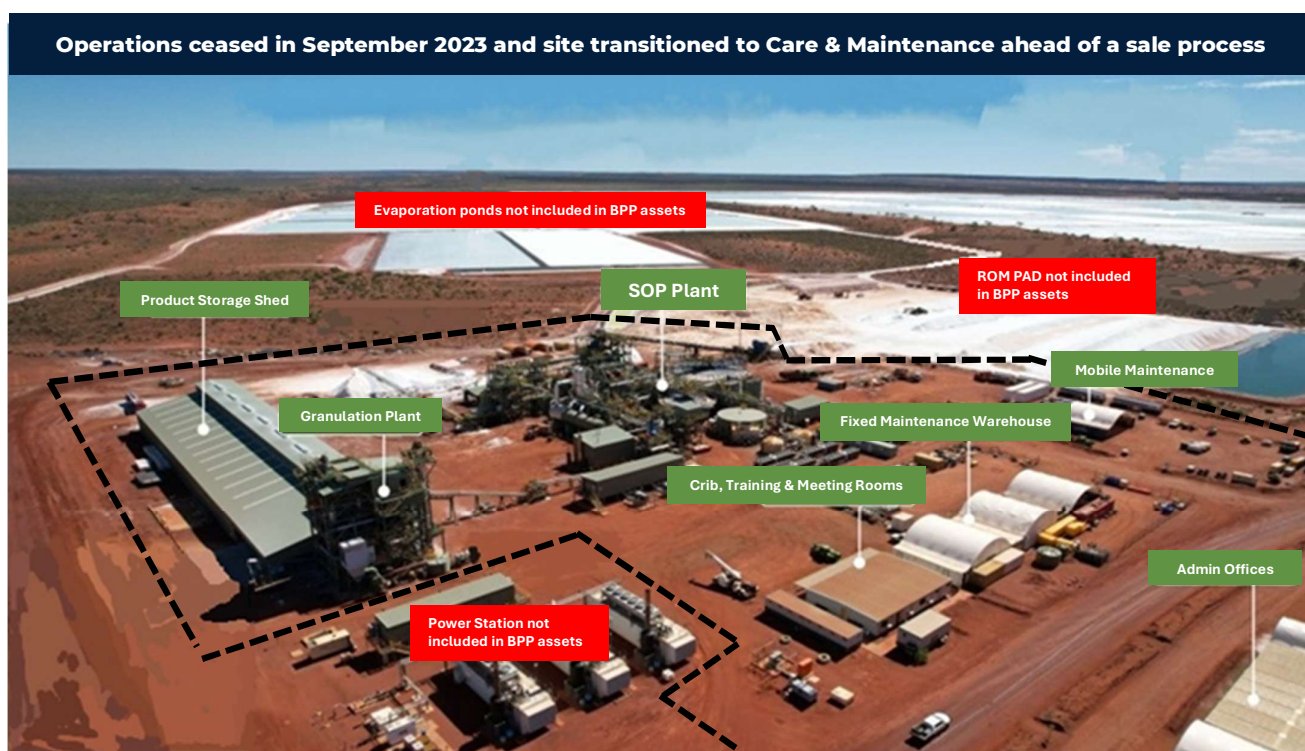
Figure 9 – Photograph of the Beyondie Potash Project in 2023 when in operation by Kalium. The Transaction comprises a fully constructed processing plant, site offices and maintenance infrastructure. Specific plant components include, KTMS crushing circuit, Kainite conversion circuit, column flotation circuit, liquor cooling heat exchangers, evaporative cooling circuit, product separation centrifuges, SOP recovery and granulation units, RO water plant and a bulk storage shed.
