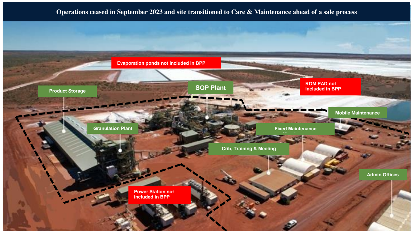
Figure 13 – Photograph of the Beyondie Potash Project in 2023 when in operation by Kalium. The assets include a fully constructed processing plant, site offices and maintenance infrastructure. Specific plant components include, KTMS crushing circuit, Kainite conversion circuit, column flotation circuit, liquor cooling heat exchangers, evaporative cooling circuit, product separation centrifuges, SOP recovery and granulation units, RO water plant and a bulk storage shed. 1
