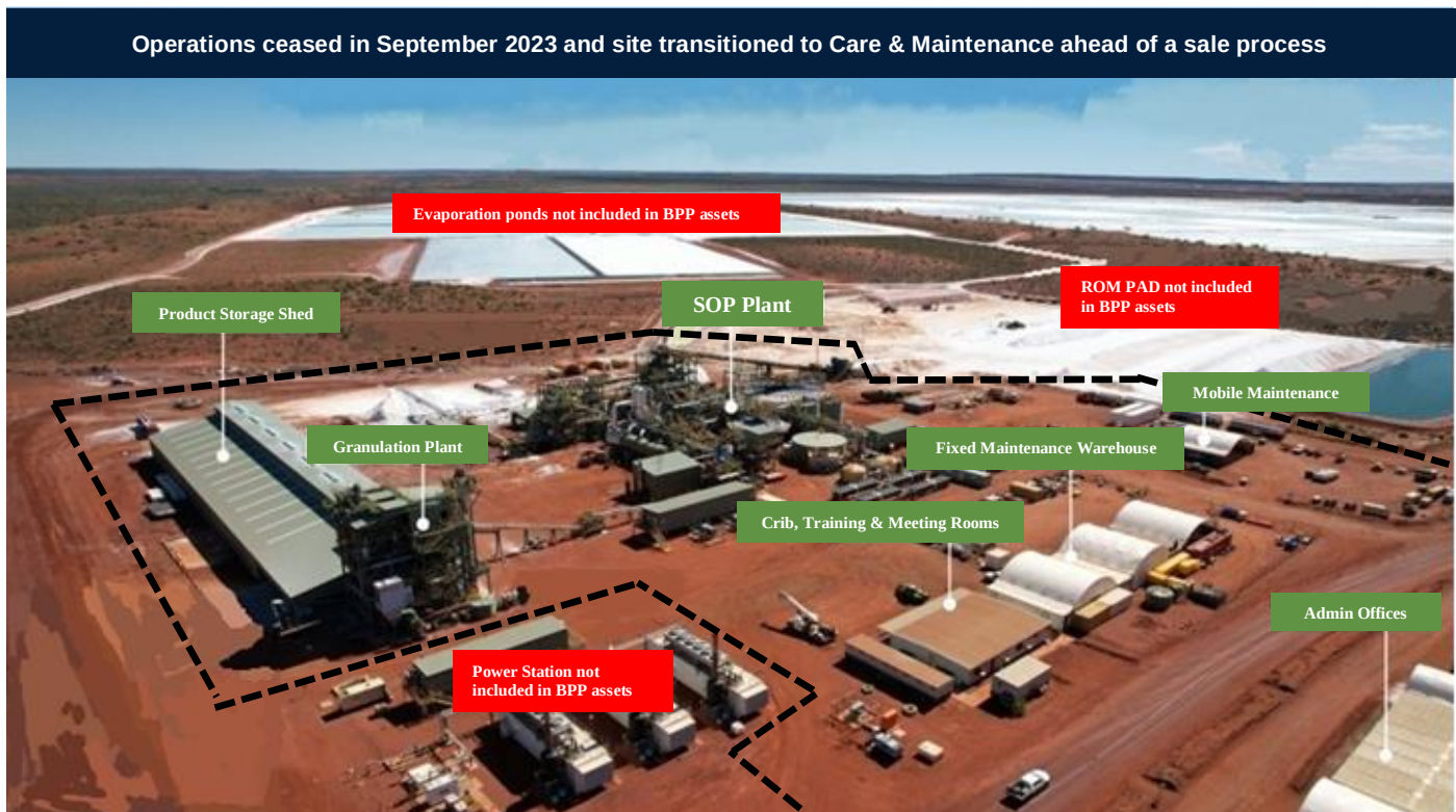
Figure 9 – Photograph of the Beyondie Potash Project in 2023 when in operation by Kalium Lakes Ltd (Kalium). The assets include a fully constructed processing plant, site offices and maintenance infrastructure. Specific plant components include, KTMS crushing circuit, Kainite conversion circuit, column flotation circuit, liquor cooling heat exchangers, evaporative cooling circuit, product separation centrifuges, SOP recovery and granulation units, RO water plant and a bulk storage shed. 1
